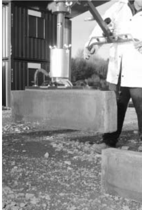
Figure 1 Handling kerbs using a vacuum lifter
